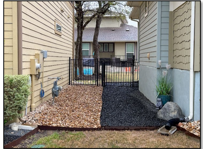
Right: Non-combustible fence attached directly to
